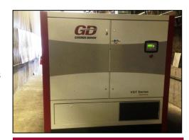
Equipment air intake openings located at foot traffic level are prone to pull in dust and debris along with necessary fresh air.
