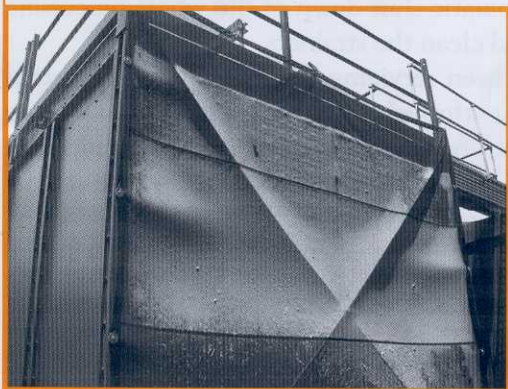
PreVent® air intake filter captures cottonwood before it enters the 650 ton Marley Cooling Tower
