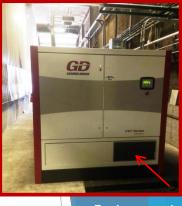
Equipment air intake openings located at foot traffic level are prone to pull in dust and debris along with necessary fresh air.
