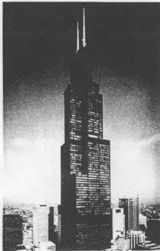
Permanent filters were installed on the 108th floor of the Sears Tower.
