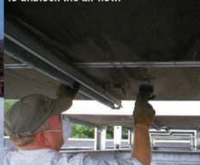
Dirty fins and coils require hand cleaning and chemicals to unblock the air flow.
