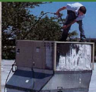
Dirty fins and coils require hand cleaning and chemicals to unblock the air flow.
